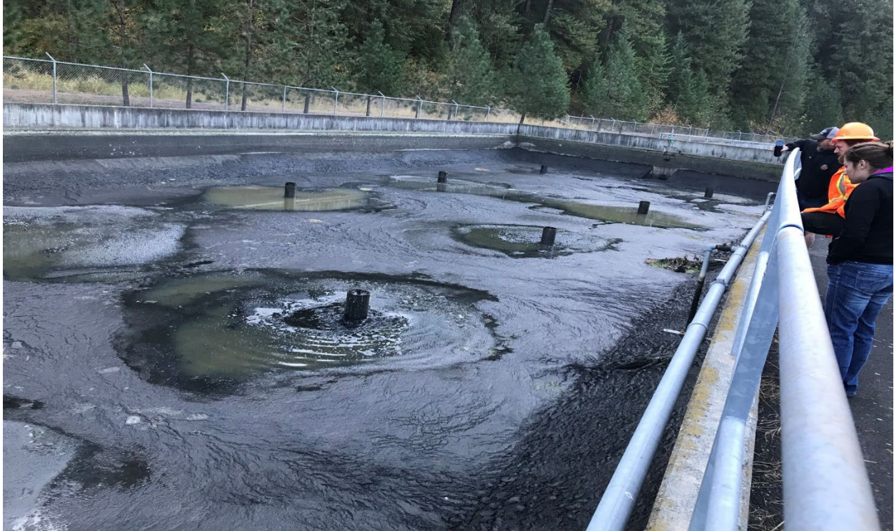
Photo 2-1: Cell 1 Prior to Solids Removal
