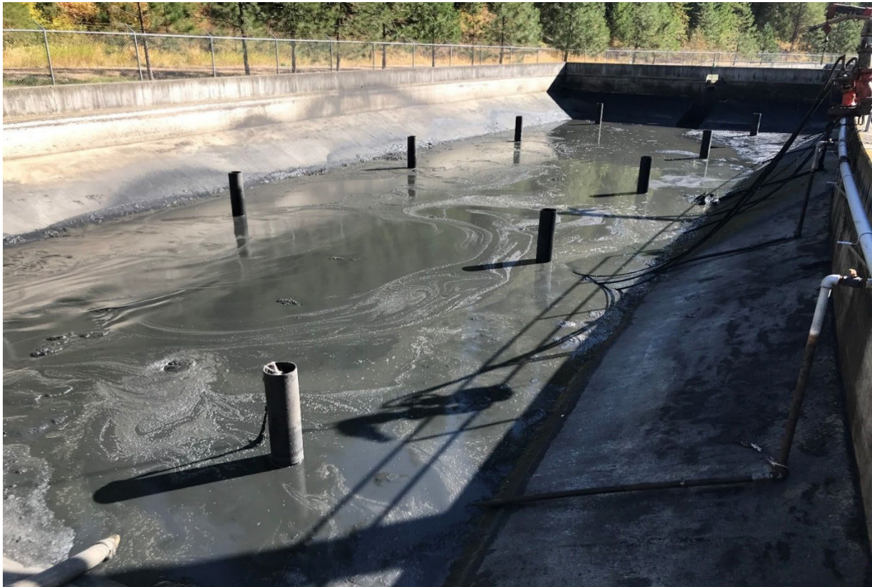
Photo 2-2: Cell 1 After Solids Removal
