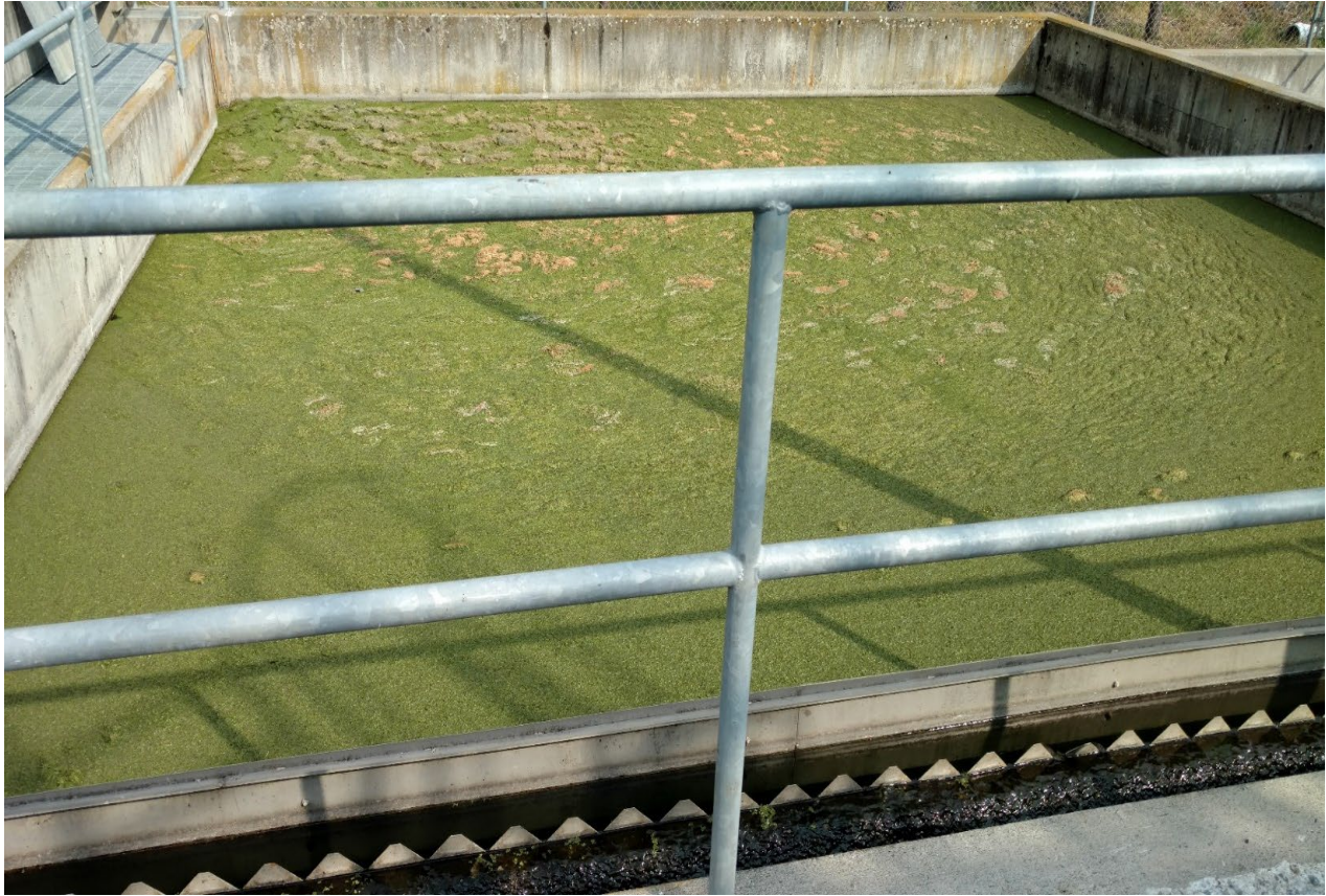
Photo 2-5: Cell 4 During Summer
